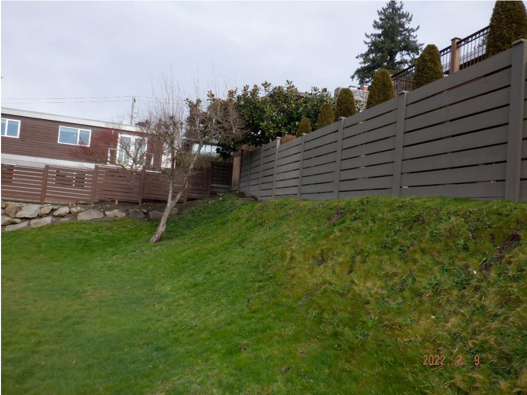
Looking north to northeast property corner
